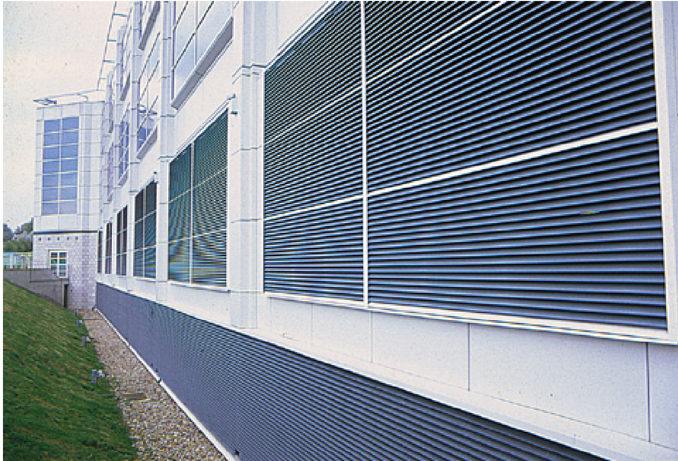
Perforated single bank louvre
